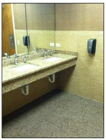
so as not to disrupt the convenience of the tenants. The project included installing new toilet partitions, new floor and wall tile, wall coverings, granite counter tops and sinks.
